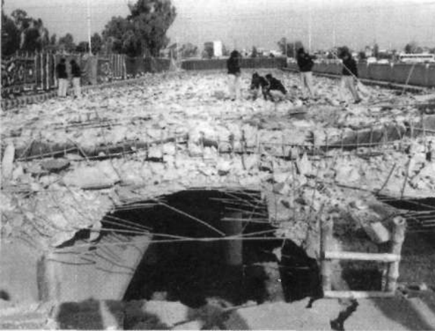
The blown-up bridge, after the assassination attempt of December 14, 2003
